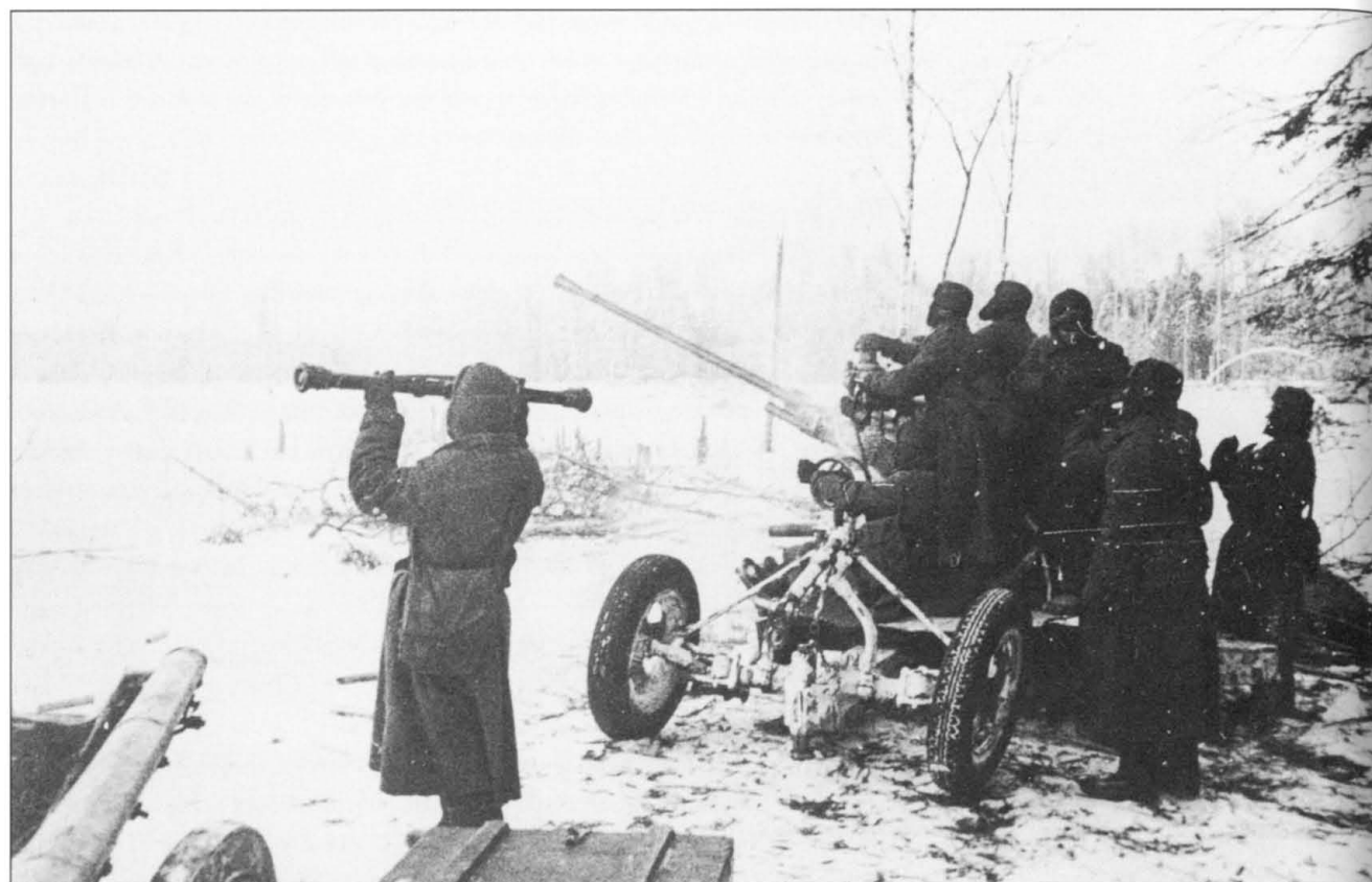
A Soviet light anti-aircraft gun waits for a clear sighting outside of Murmansk. The soldier to the left of the gun is using a range finder to determine the distance to the target.
