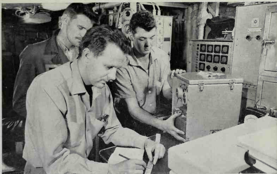
39. Checking operation of inertial navigation system, used in obtaining exact position of Nautilus under North Pole.
